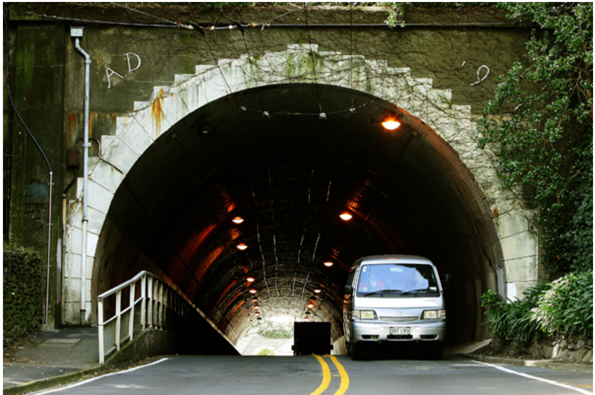
Crawford Tunnel, Seatoun, Wellington (Photo: Fairfax)
