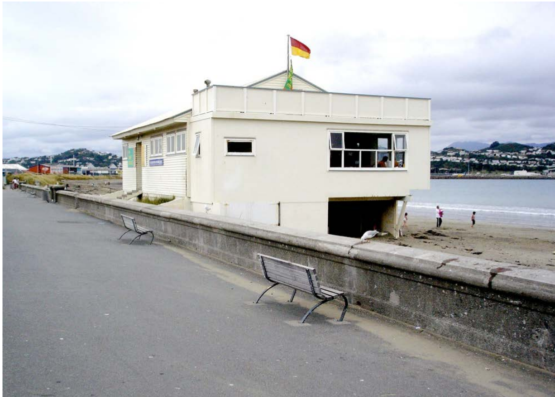
Lyll Bay Sea Wall (Photo: WCC, 2010)
