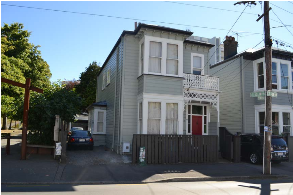
46 Aro Street – Image: Charles Collins – 2015
