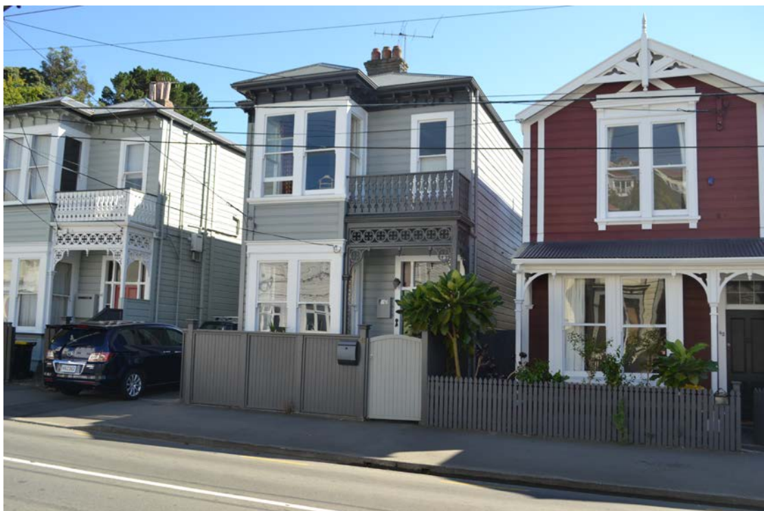
44 Aro Street – Image: Charles Collins – 2015
