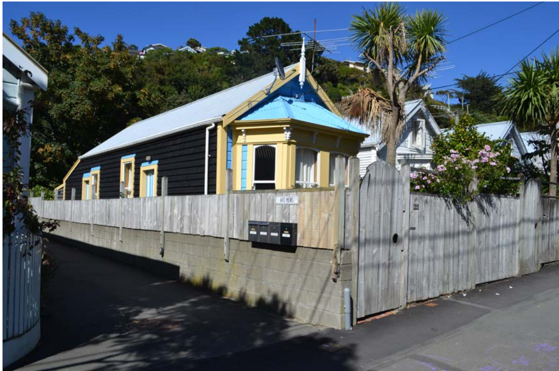
125 Aro Street – Image: Charles Collins – 2015
