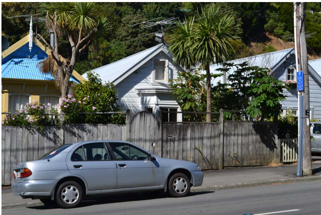
127 Aro Street – Image: Charles Collins – 2015
