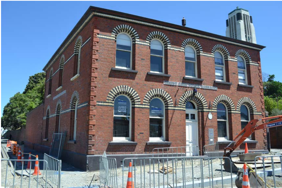
Mount Cook Police Station, Image: Charles Collins, 2015
