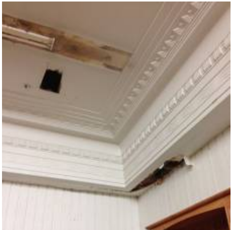
Deka Building interior in 2012. Image: WCC ref 2012 June Cuba 004
