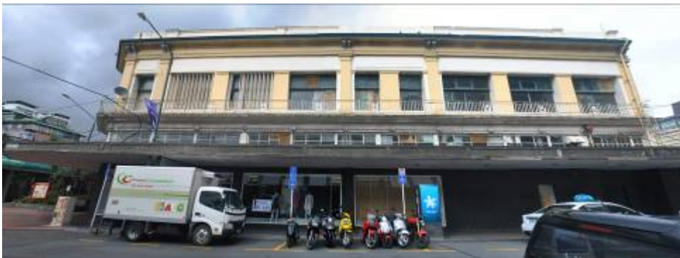
Merged photograph to show the Ghuznee Street Elevation. Image: WCC taken 11 November 2011, reference 11nov2011- 11
