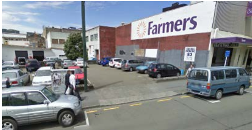
North elevation of the rear (probably circa 1962 building) from Victoria Street. Image: Google Maps - ©2012 image 2009
