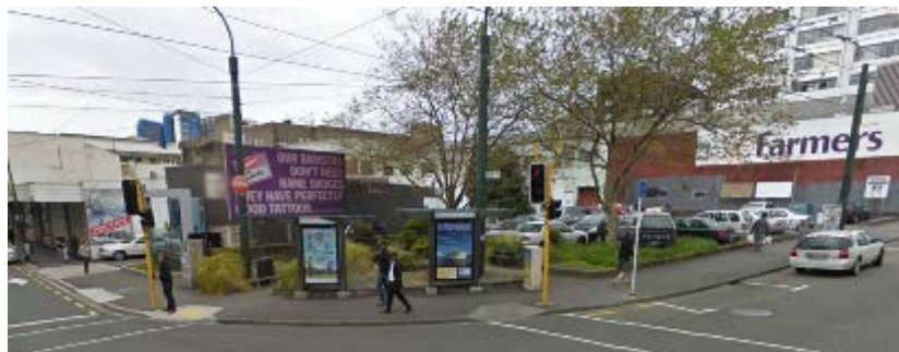
North elevation from the corner of Dixon and Victoria Streets of the rear (probably circa 1962 building). Image: Google Maps - ©2012 image 2009
