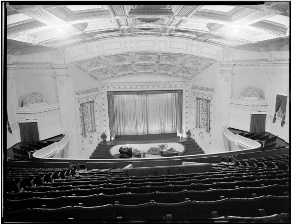
Interior of the Embassy Theatre, Wellington, looking towards the stage, ca 1925, Reference Number: 1/1-015962-F, accessed May 2013, at http://mp.natlib.govt.nz/detail/?id=4323
