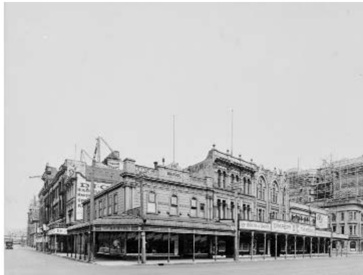
1927 Lambton Quay, Wellington, with premises of the Bristol Piano Company and the DIC. ID: 1/4-014992-F
