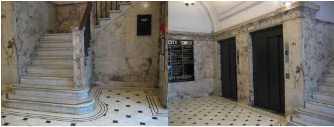
Panama Street lobby (2012). Images: WCC ref 7296 & 7298
