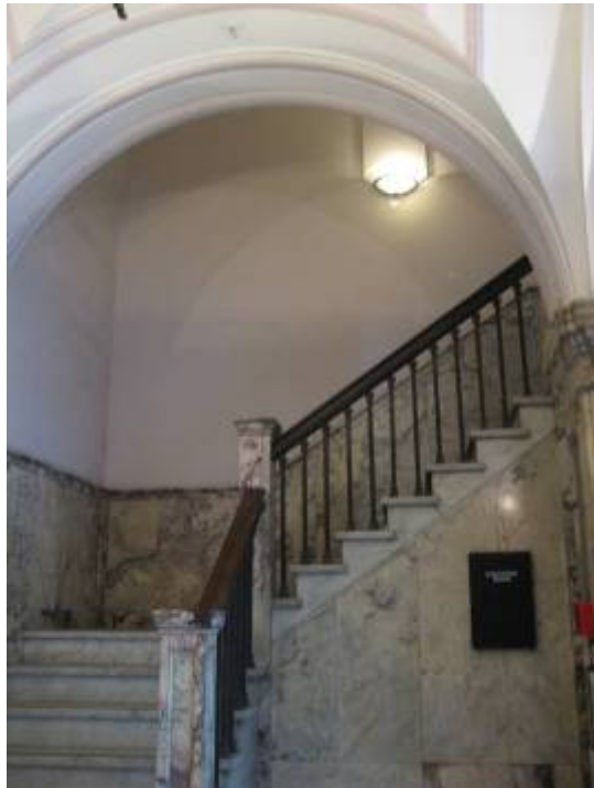
Panama Street lobby (2012). Images: WCC ref 7297
