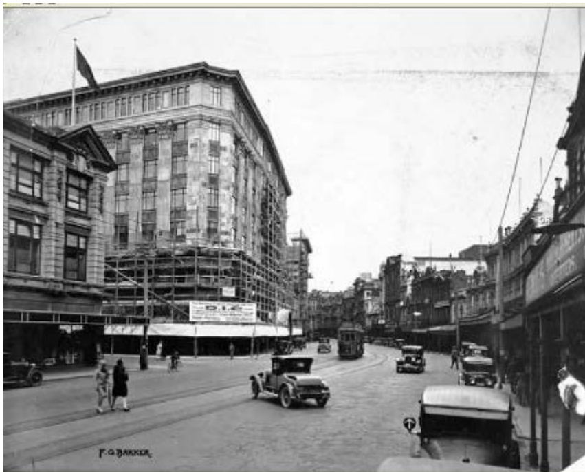
1928 Newly constructed DIC department store, Lambton Quay between Panama Street and Brandon Street, Scaffolding has not yet been removed. Image: FG Barker WCC Archives 00138_0_11042
