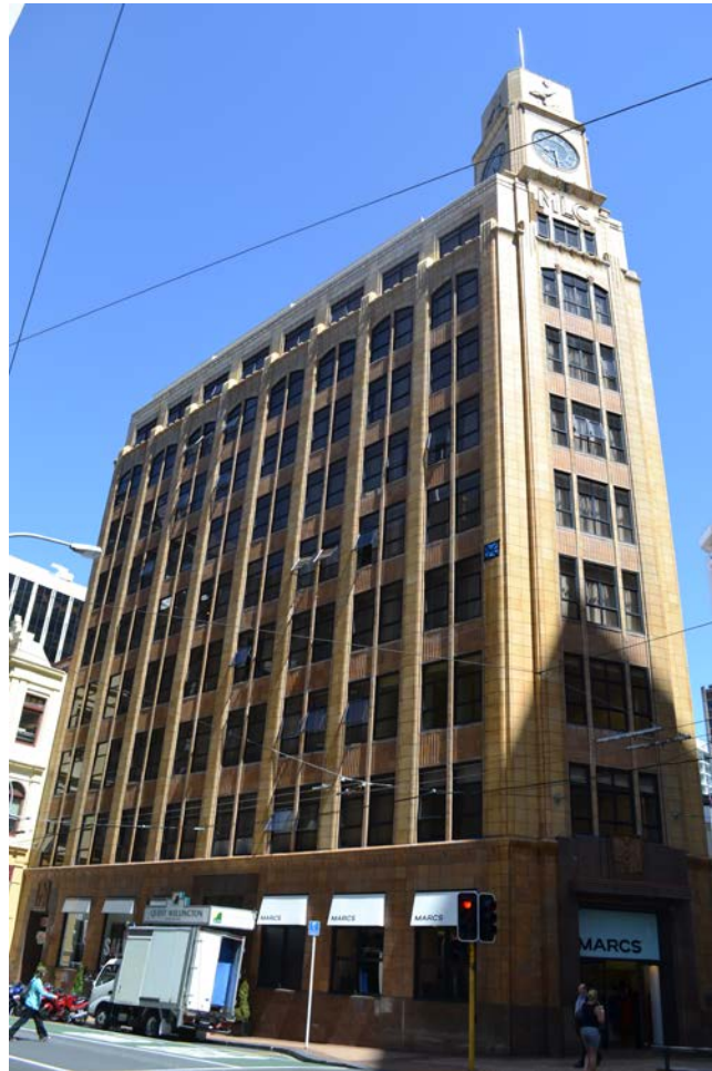
MLC Building, 231 Lambton Quay (Photo: Charles Collins, 2015 )
