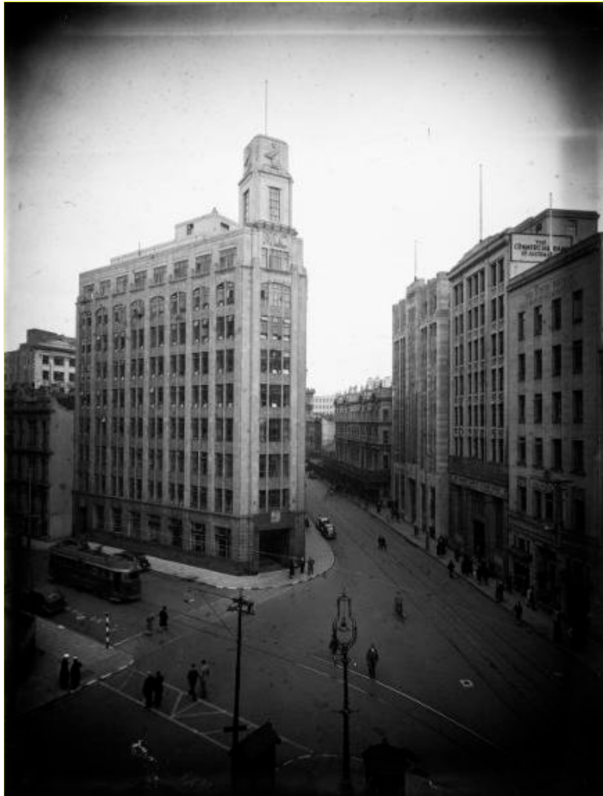
c.1940 Photograph of the MLC Building before the installation of the clock and bells 3
