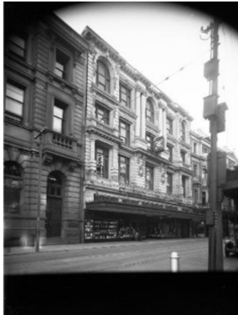
Whitcombe and Tombs Ltd, c1940. Note that the decorative parapets/entablature were removed in 1935 before this photograph was taken, they have since been replicated in lightweight materials. (ATL 1/1-021947)
