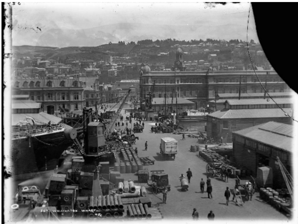
c.1900 image of Shed 3 prior to the second storey addition. 7
