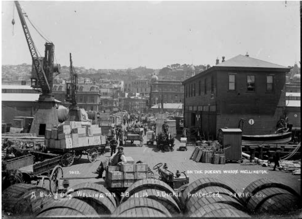
1913 image of Shed 3 with the second floor addition. 8
