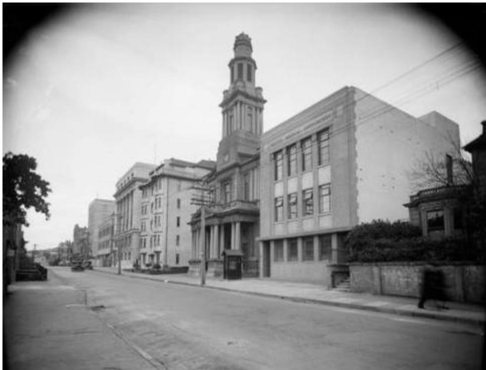
View of the BMA Building (foreground), with St Andrews and Braemar to the left, c1930s.
