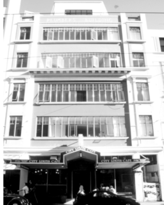
The building c2000. Note the 1995 penthouse addition visible above the parapet (2001 Inventory).
