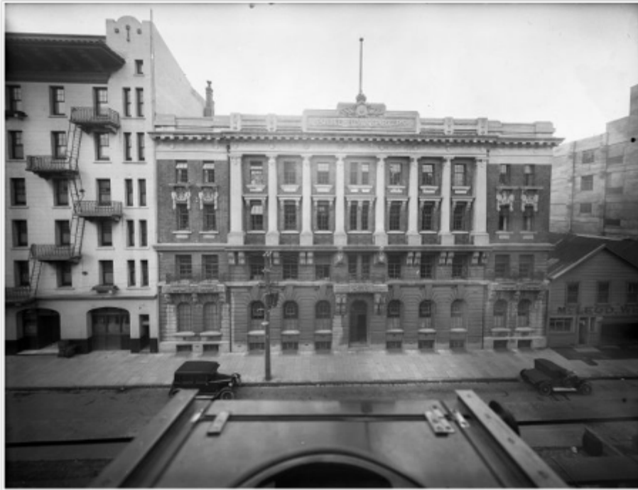
1920s photograph of the Johnston Street entrance to the Police Headquarters 16
