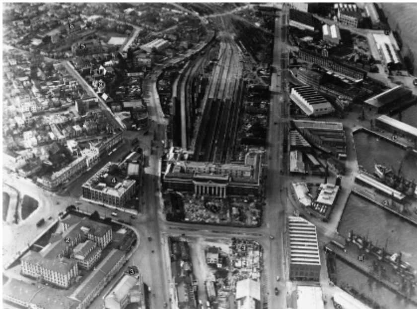
Maritime House and Shed 35. 5
