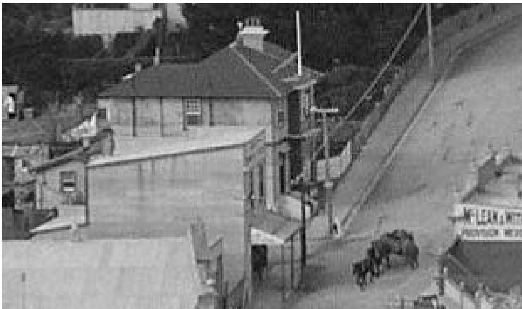
Enlarged part of previous photograph to show the Post Office building at the intersection of Cleveland and Jefferson Streets.
